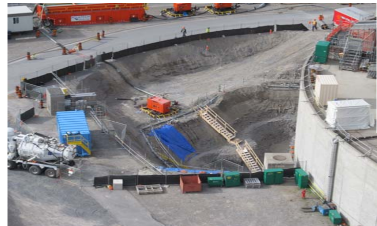
Containment Filter Venting System Construction Site
