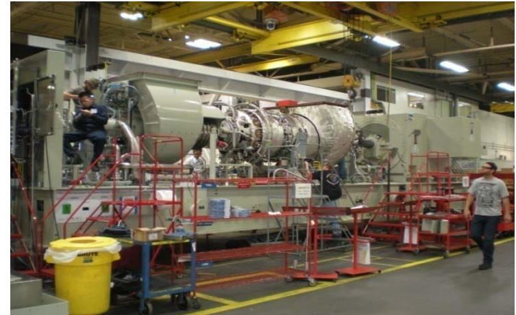
Third Emergency Power Generator
